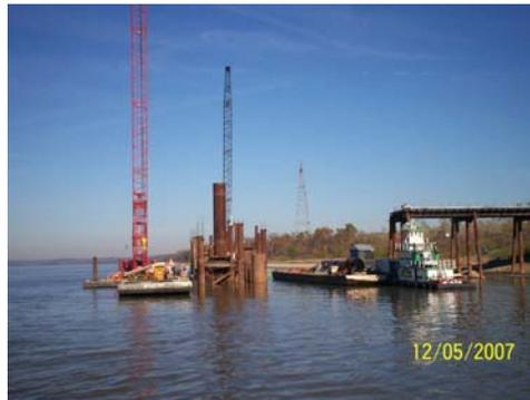
*The work trestles, when complete, will allow crews to work on the main span bridge regardless of the river conditions.*
